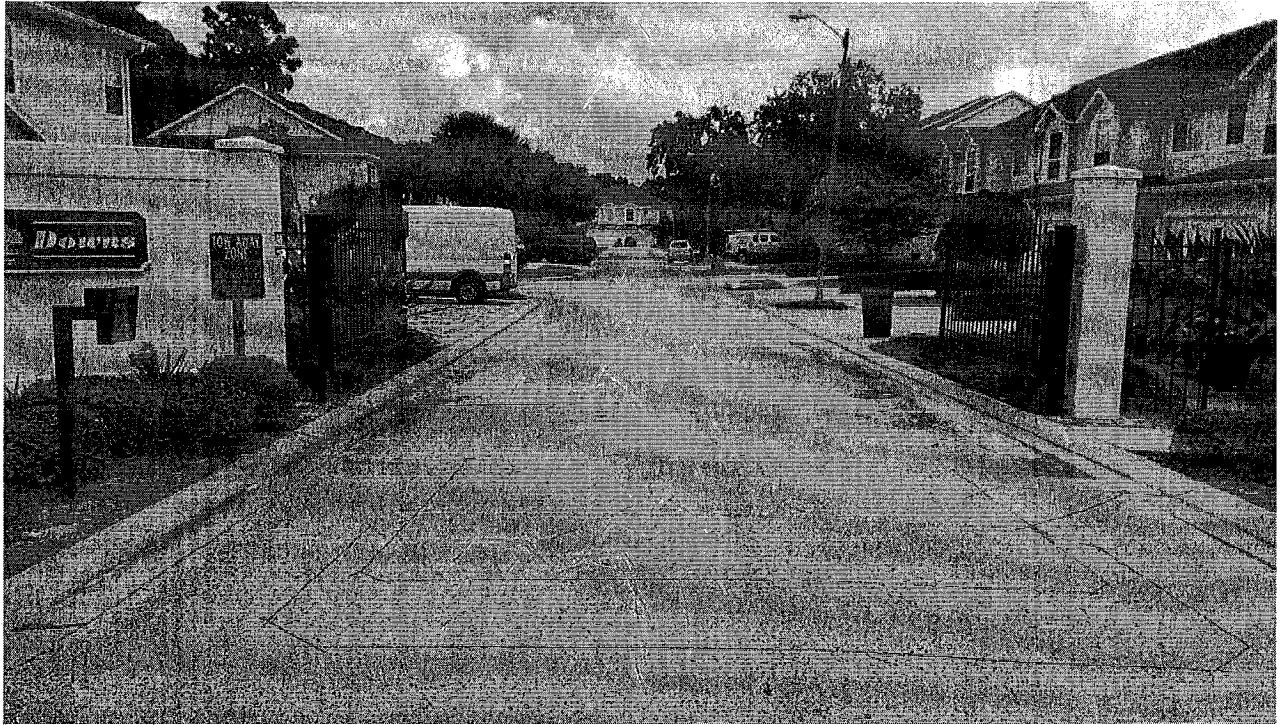
Vehicular Gate Access
